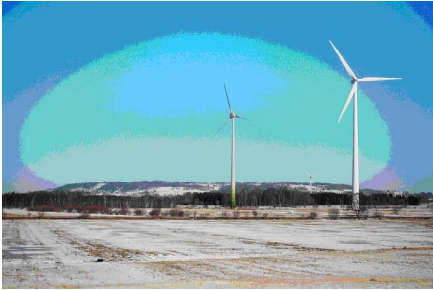
Figure A2. Examples of wind turbines that are located in a place with little risk of collision for bats and birds. They stand on level ground, well away from the height (Älleberg) and outside the obvious hinge lines. The picture was taken near Falkirk in Västergötland. Photo by Jens Rydell.
